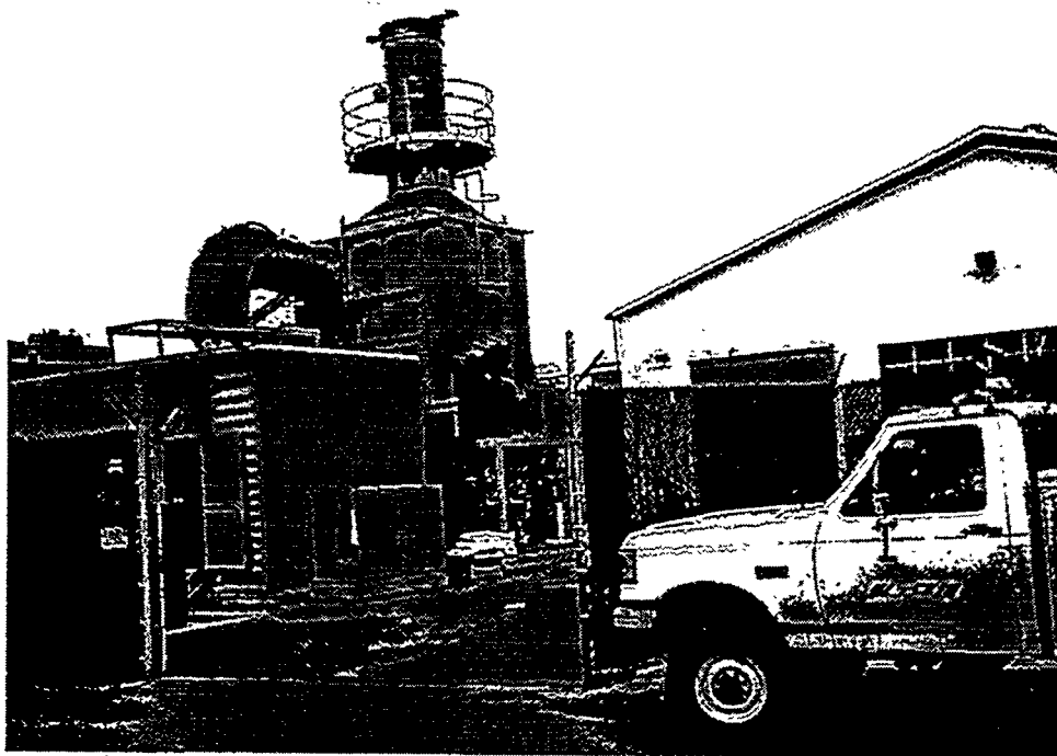
2.8 MW system established NOxTECH as BACT for diesel generators
