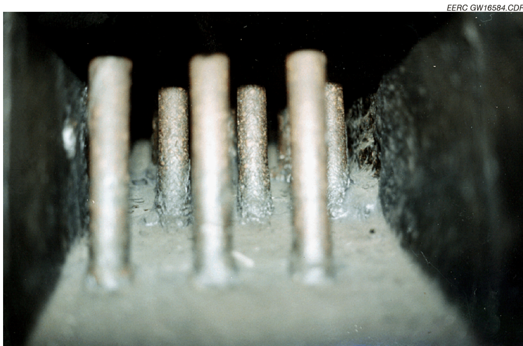
Figure 3-13. Photograph of slag screen tubes following the April test.
