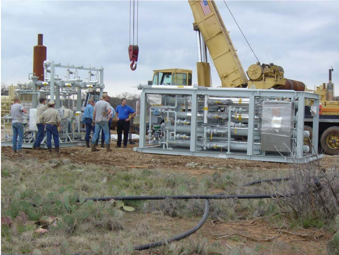
Figure 3. Membrane system being installed at Green Ranch, Texas.
