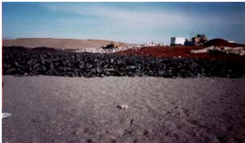
Image 6-1: Shredded tire operations layer
