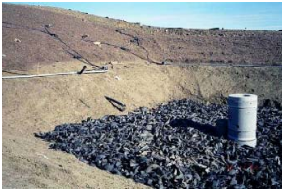
Image 5-5: Aerobic sump installed and ready for backfill
