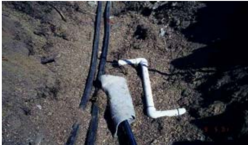
Image 5-4: Moisture, temperature, and tube installation
