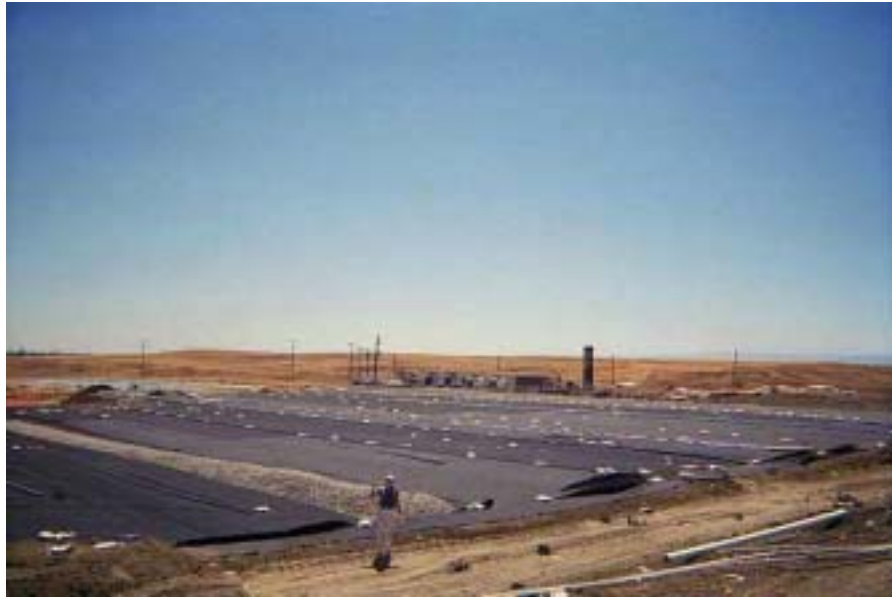
Image 5-1: Aerobic liner ready for shredded tire operations layer and waste placement
