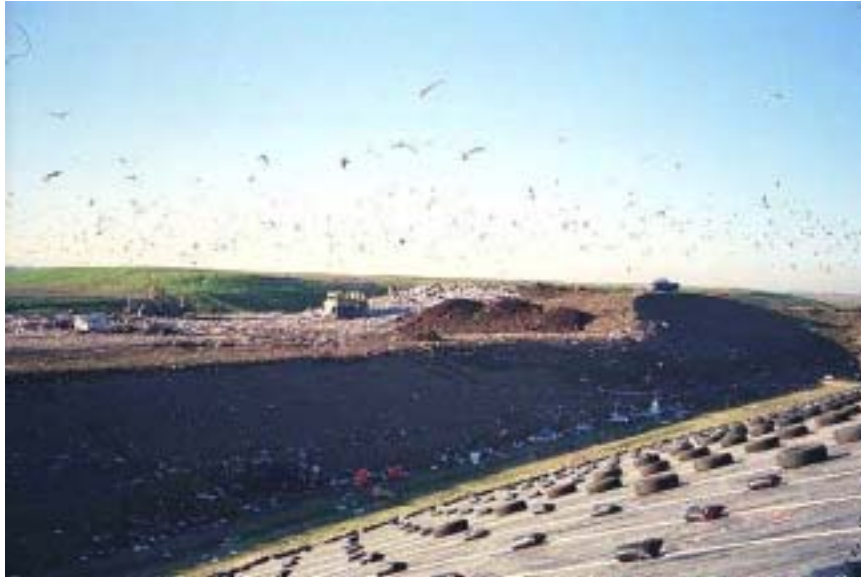
Image 4-1: Waste placement in the west-side cell
