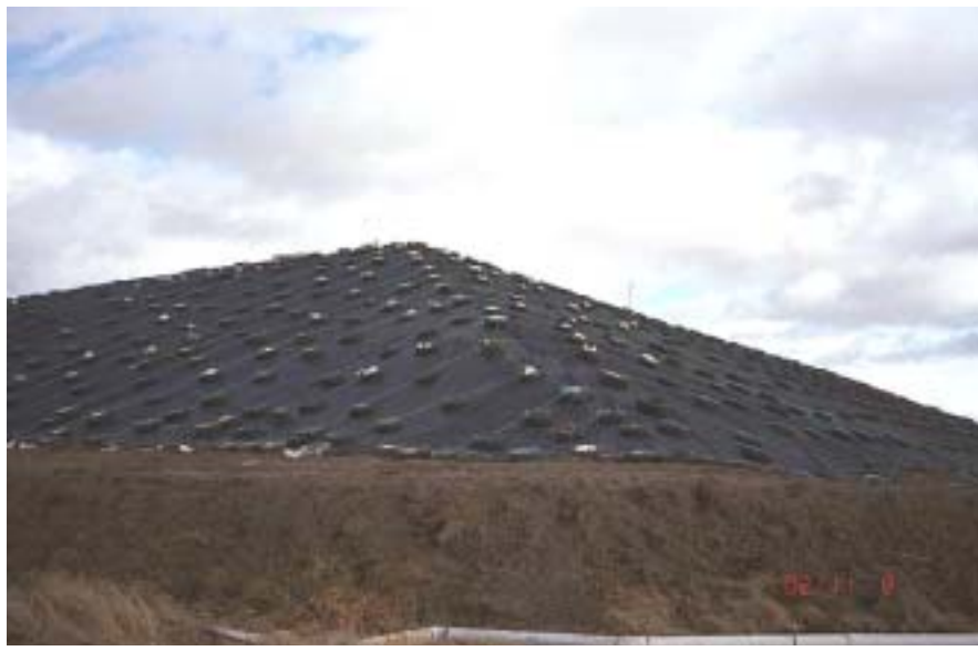
Image 4-2: West-side anaerobic cell surface liner.
