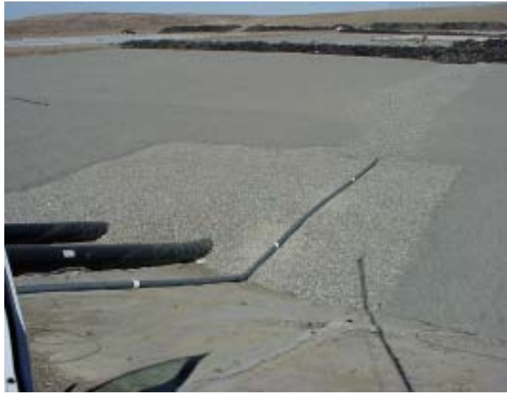
Image 3-5: Gravel drainage layer and leachate collection sump
