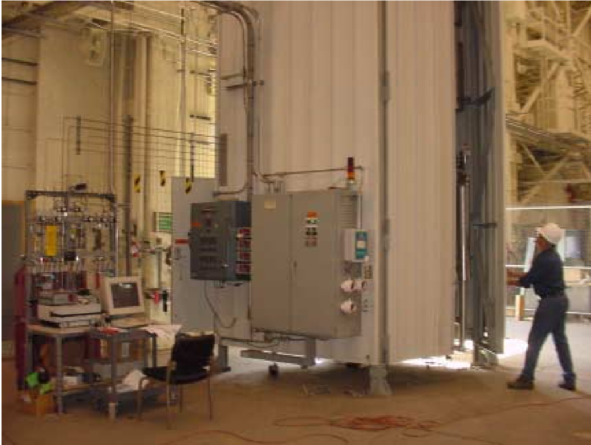
Long Tube Tester Pilot Plant Facility
