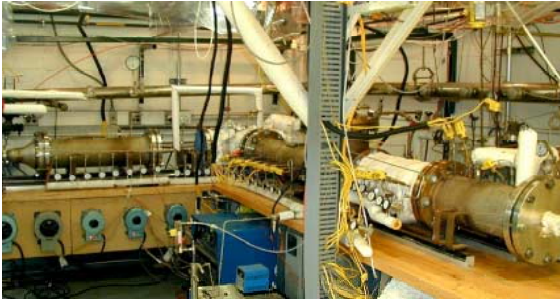
Nuvera MPR Facility: Pre-heat, Reforming, Shift and CO Cleanup Modules
