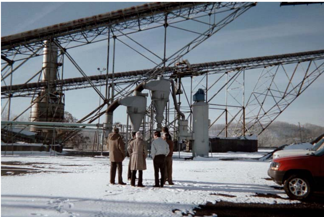
Figure 4. Existing Conveyors and Material Storage Area
