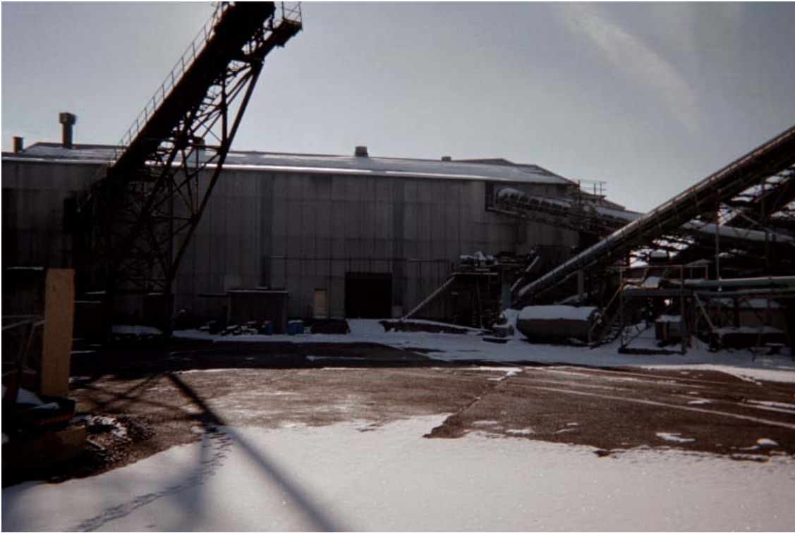
Figure 3. Old Preparation Plant to be Demolished
