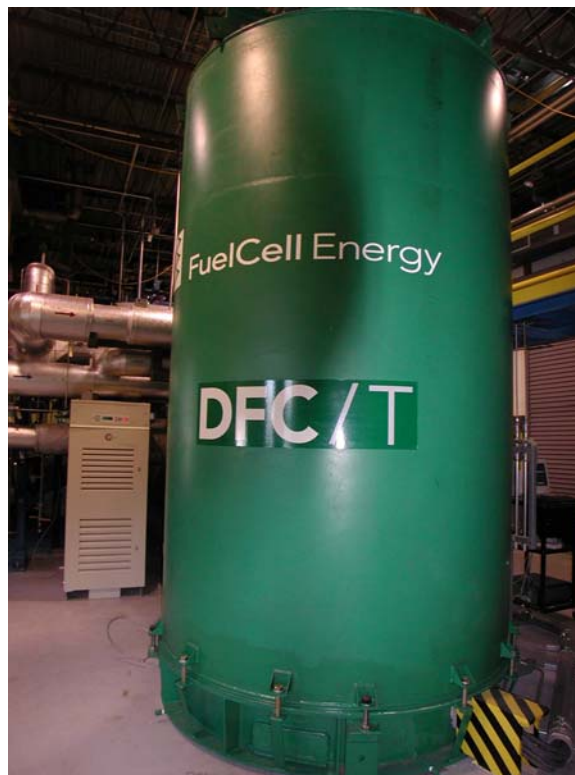
Figure 1. subMW DFC/T Hybrid Power Plant Integrated with Capstone C60
