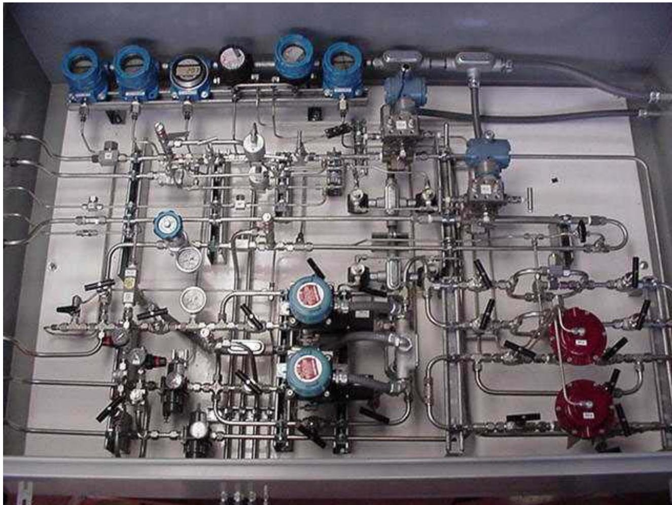
All instrument air control and nitrogen tubing are shown above. The lower left tubing is the inlet tubing and the upper left being the outlet tubing to the pyrometer camera and sight tube. The red control valves on the lower right are used to control nitrogen flowrates. The top blue displays are for various pressures and flowrates.
