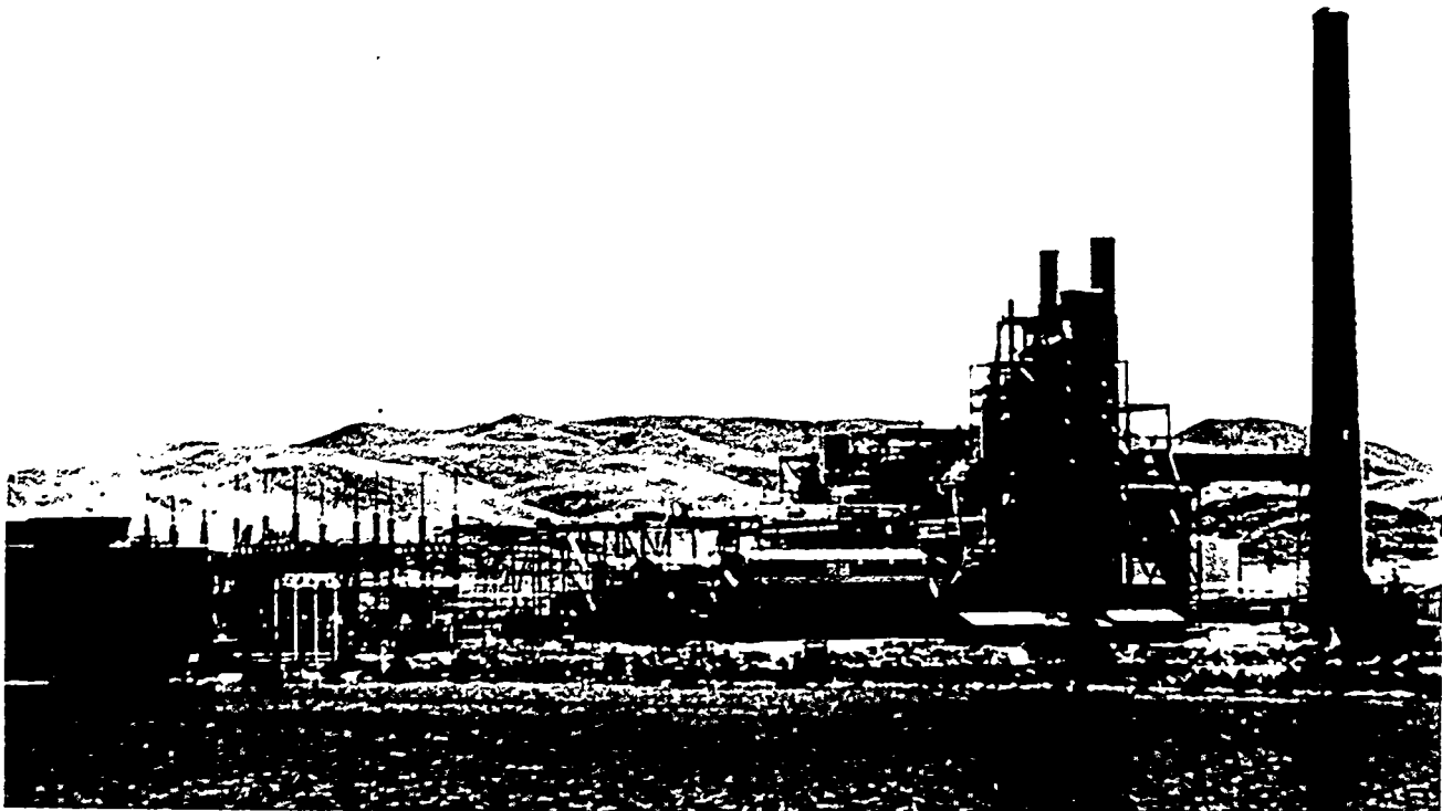
Existing steam electric units. Photo looking southeast across cooling pond for Tracy Units No. 1 & No. 2.
