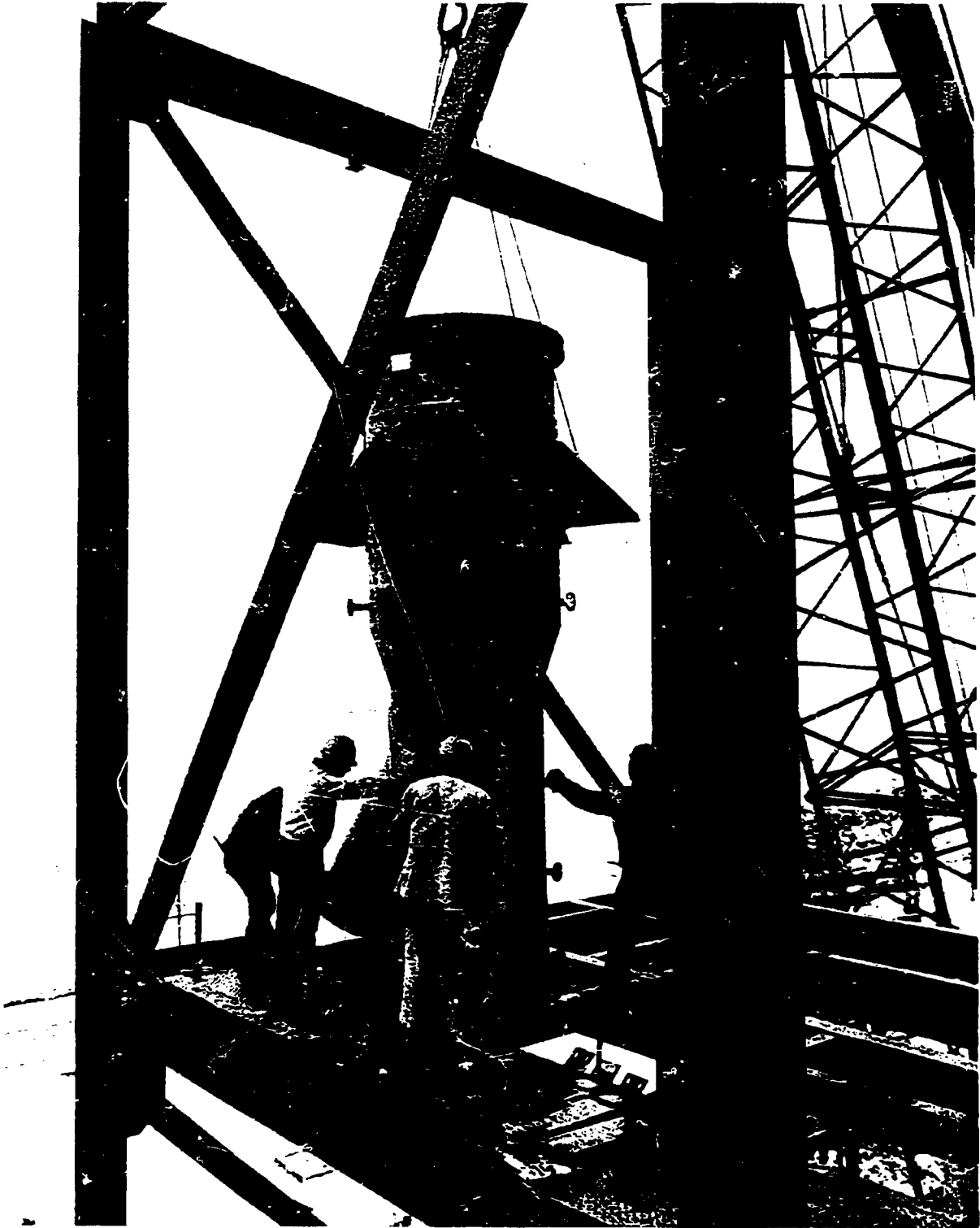
FIGURE 1. COMBUSTOR VESSEL BEING INSTALLED IN THE STRUCTURE
