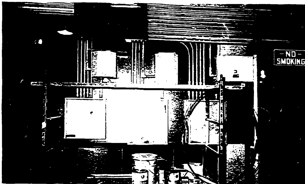
Figure 208. New Lighting Panels and Conduit
