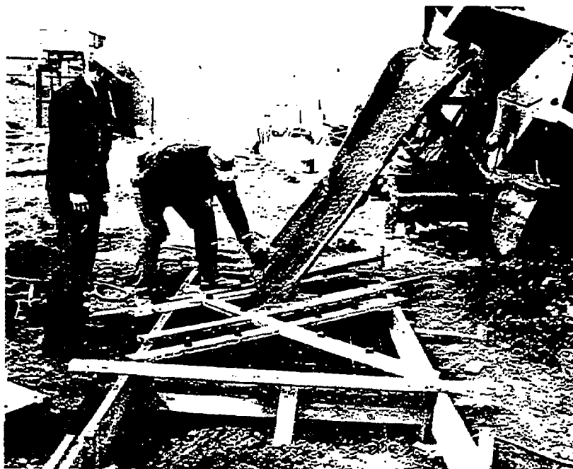
Figure 173. Pouring the Thermal Oxidizer Pad
