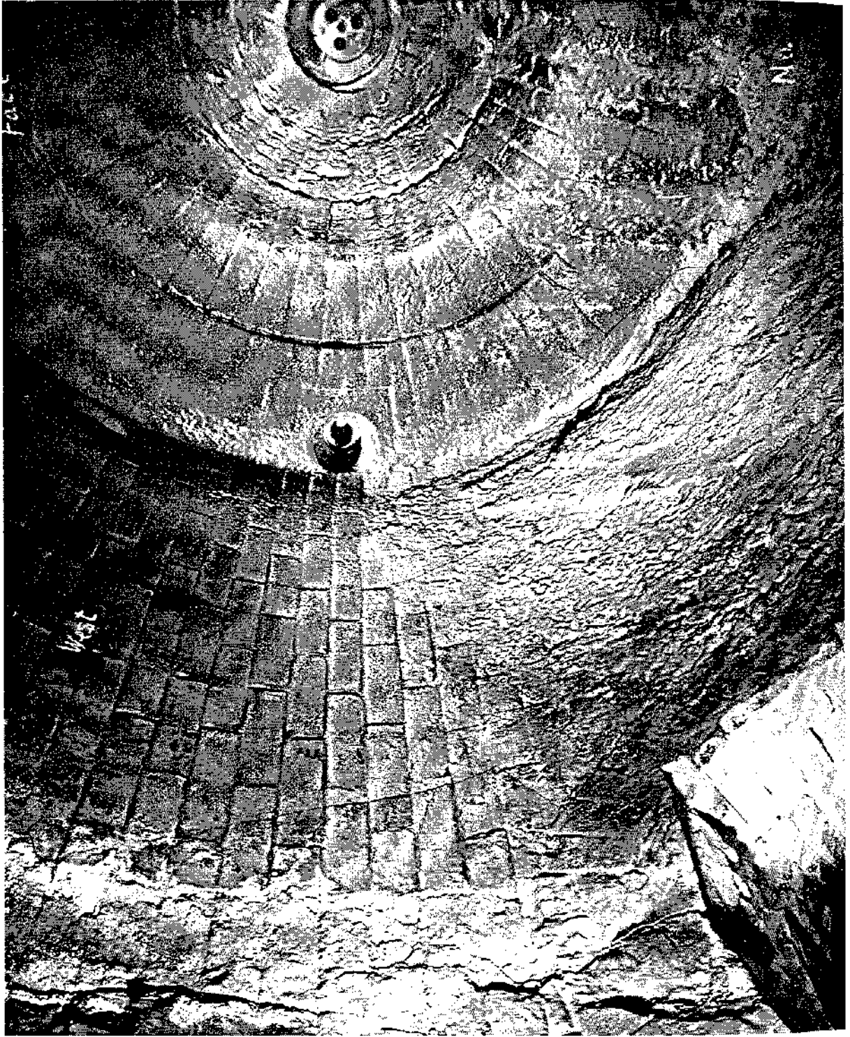
Figure 23. - Cylindrical section of gasifier, northwest view.
