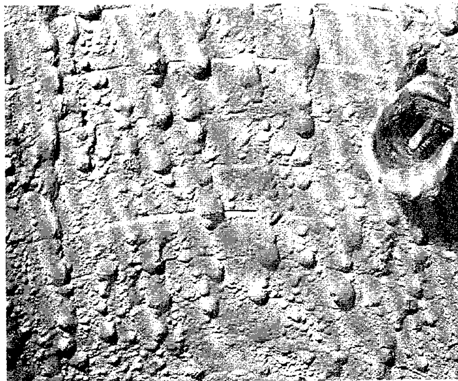
Figure 30B. - Typical slag formation on generator wall, September 1949.
