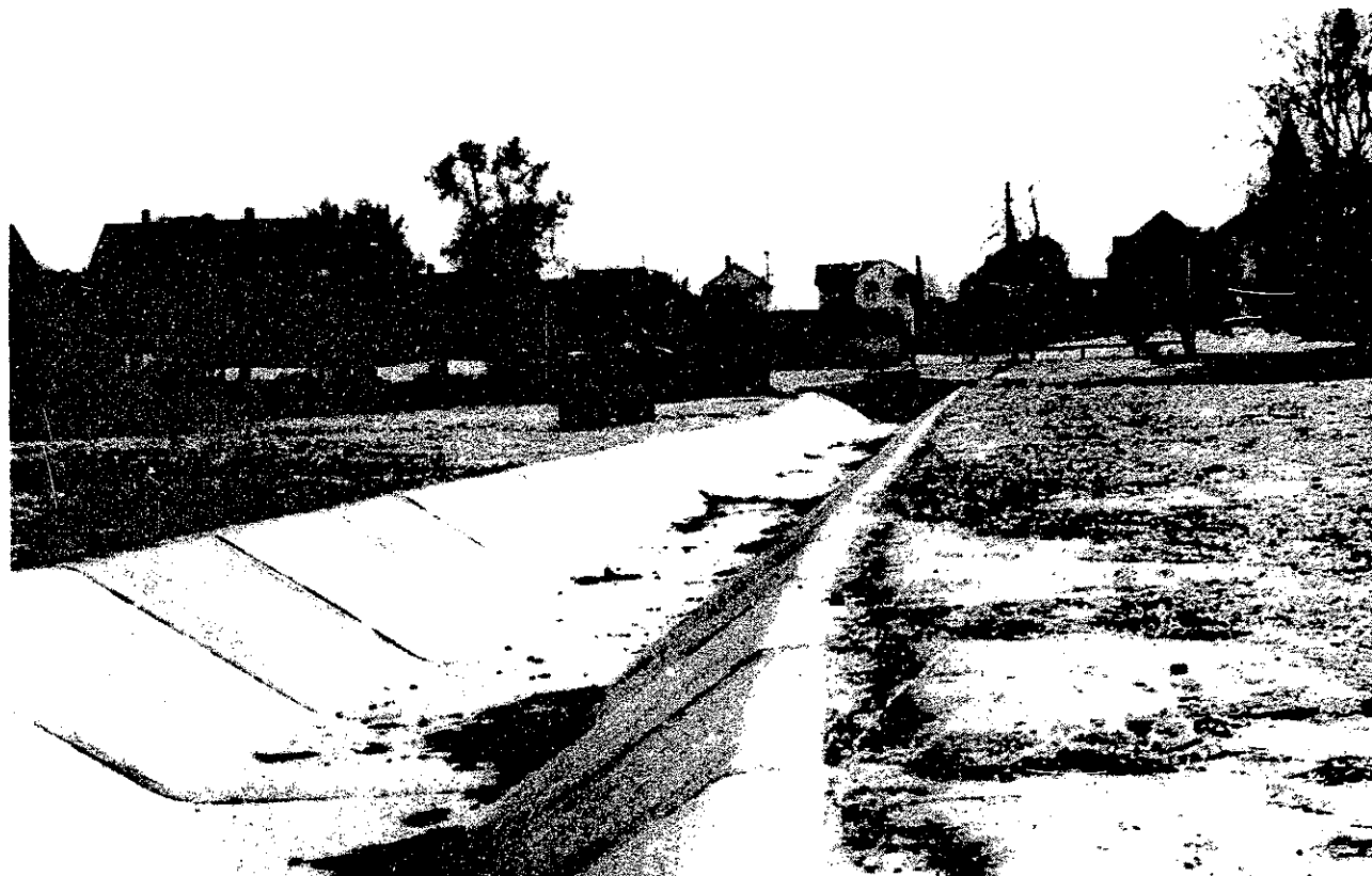
FIGURE 3. - Improvement of Stream Bed, Boston Creek, Larksville, Pa.
