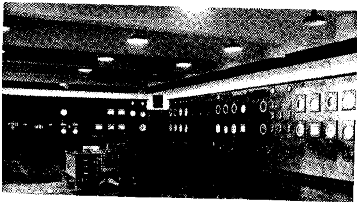
Figure 8. - Vapor-phase instruments in high-pressure control house.
