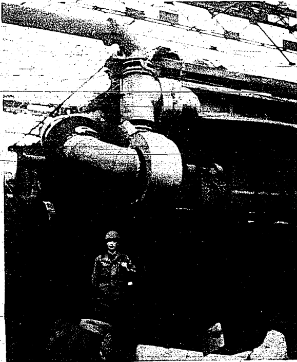
Photograph 2 Rotary Residue Kiln
