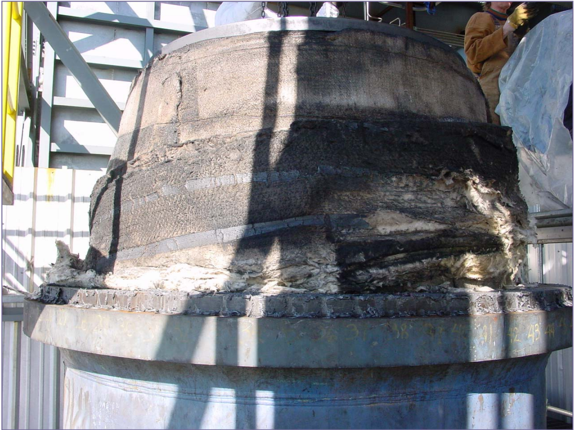
Figure 3.3-8 Clean Side of Tubesheet
