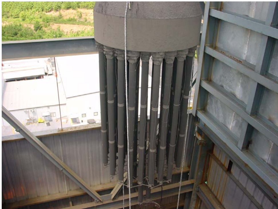
Figure 3.3-10 PCD Internal Removal (Lower Plenum)
