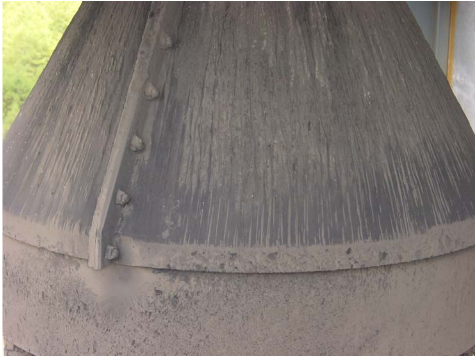
Figure 3.3-11 G-ash Accumulation on Top Ash Shed
