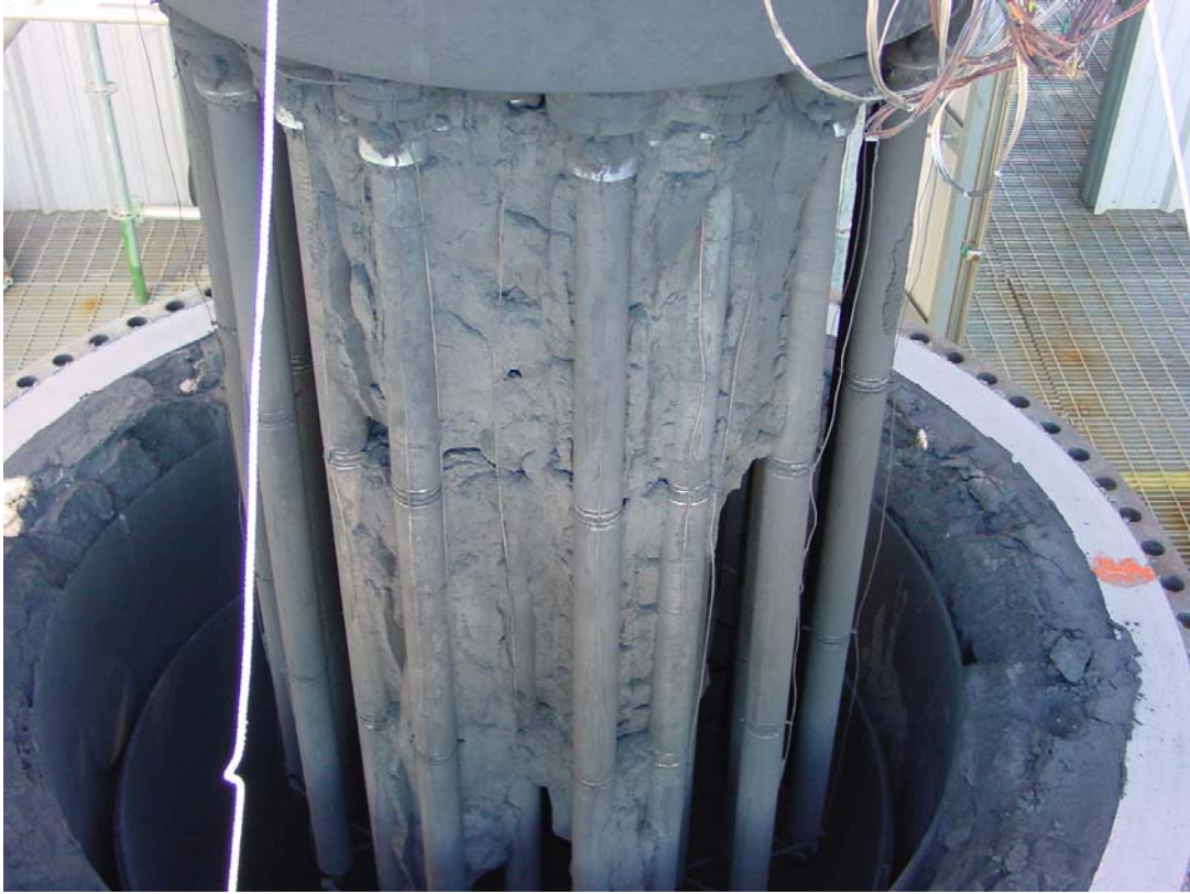
Figure 3.3-15 Removal of PCD Internals After TC06B
