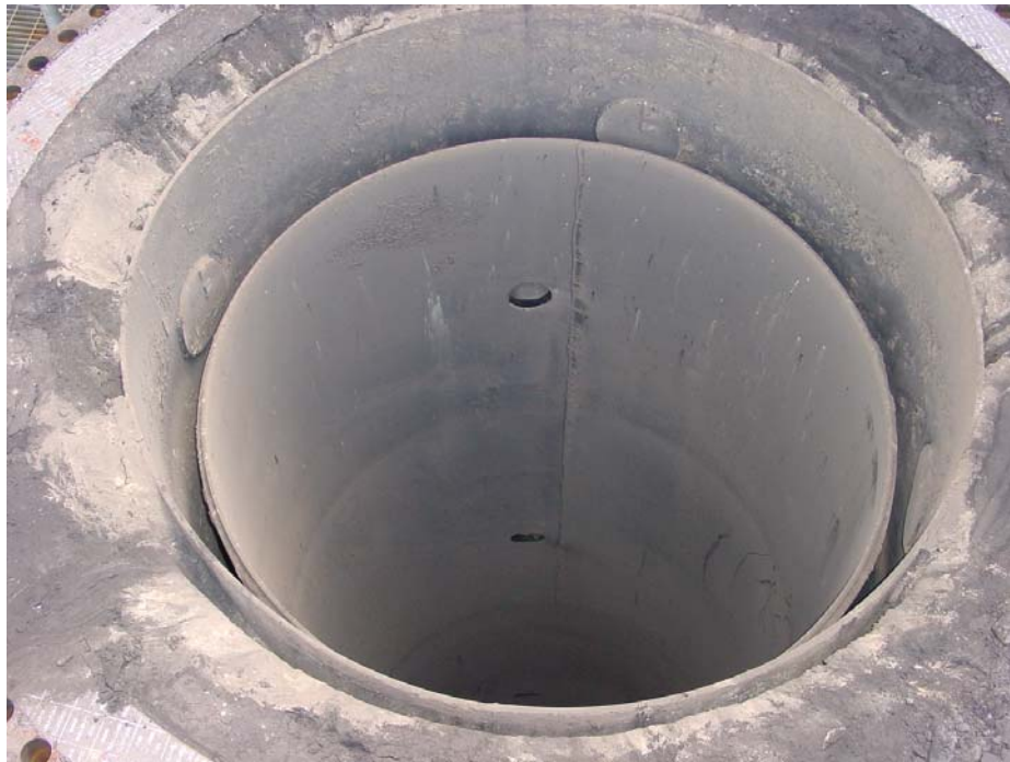
Figure 3.3-12 PCD Internal Shroud and Liner
