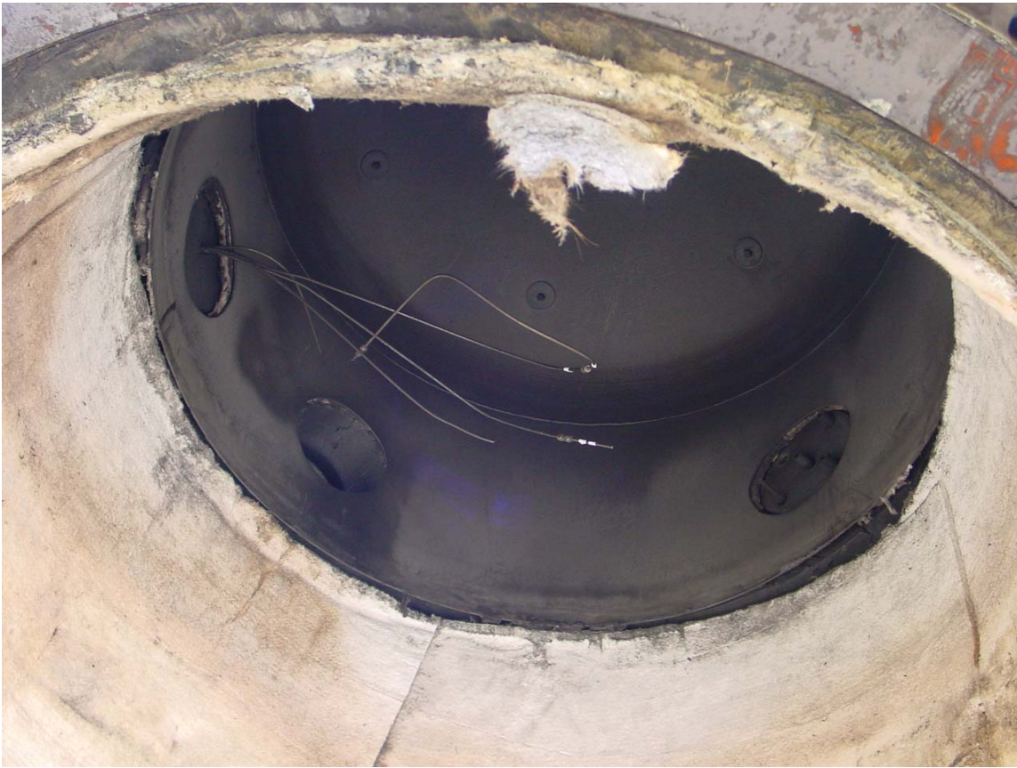
Figure 3.3-25 PCD Head Insulation
