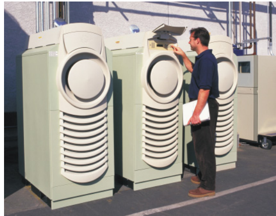
Three 30-kW microturbines are in use at a landfill in Burbank, California, to generate electricity.
