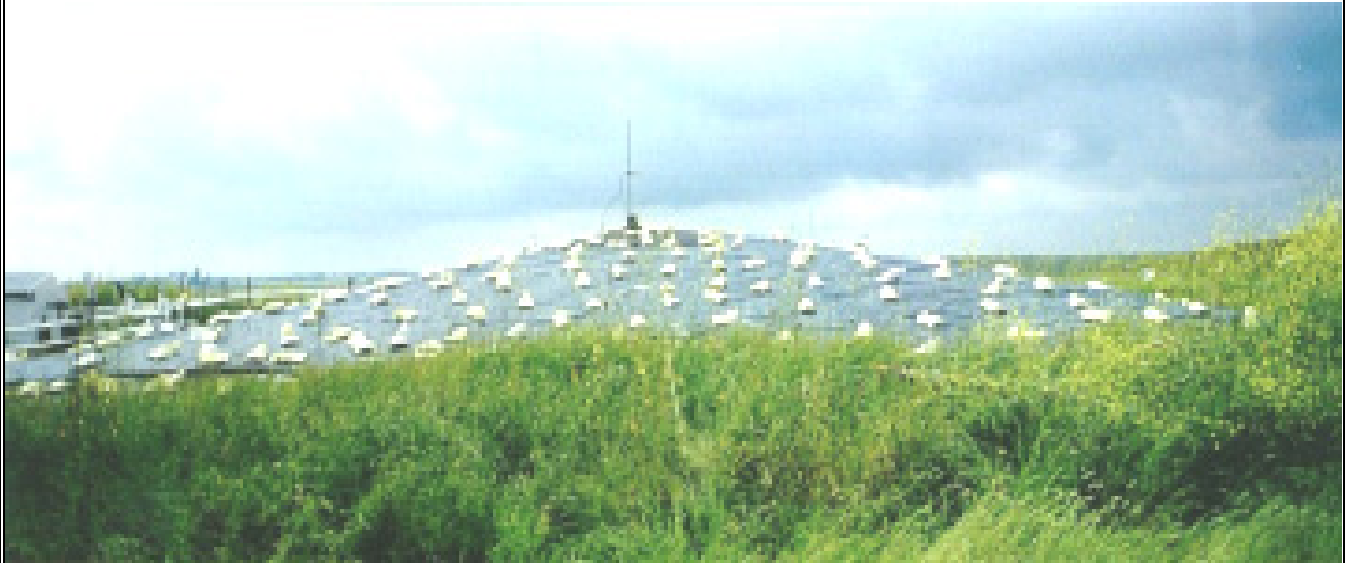
Landfill bioreactor cell, Yolo County, California
