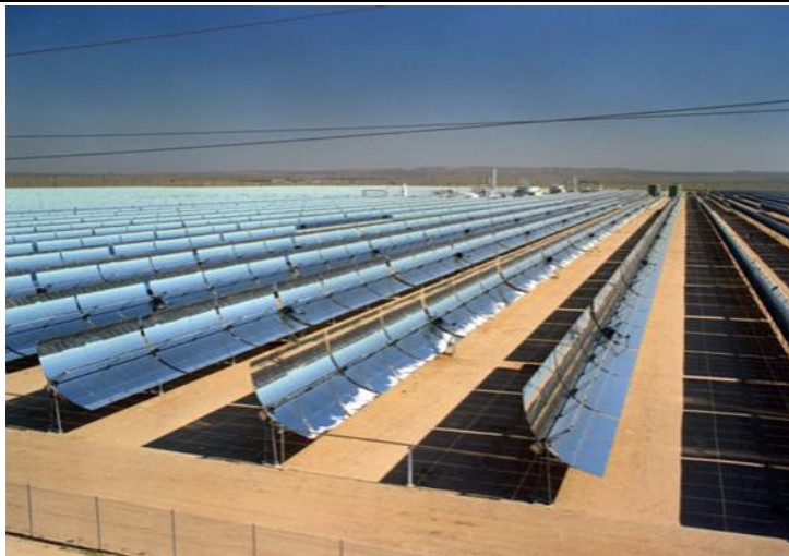
Luz Trough Power Plant
