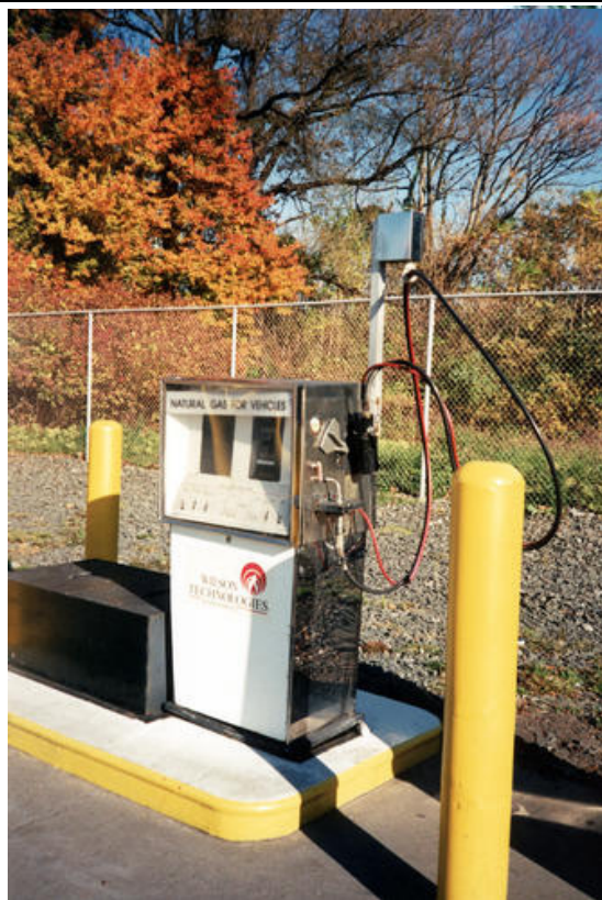
A school bus in New Jersey runs on biodiesel (right). United Parcel Service maintains a natural gas compressor station and CNG fueling island at several facilities in Connecticut (left).
