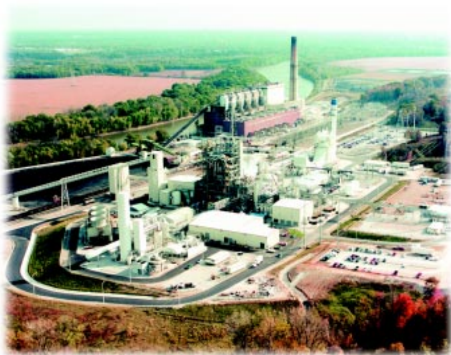
Wabash River Coal Gasification Repowering Project
