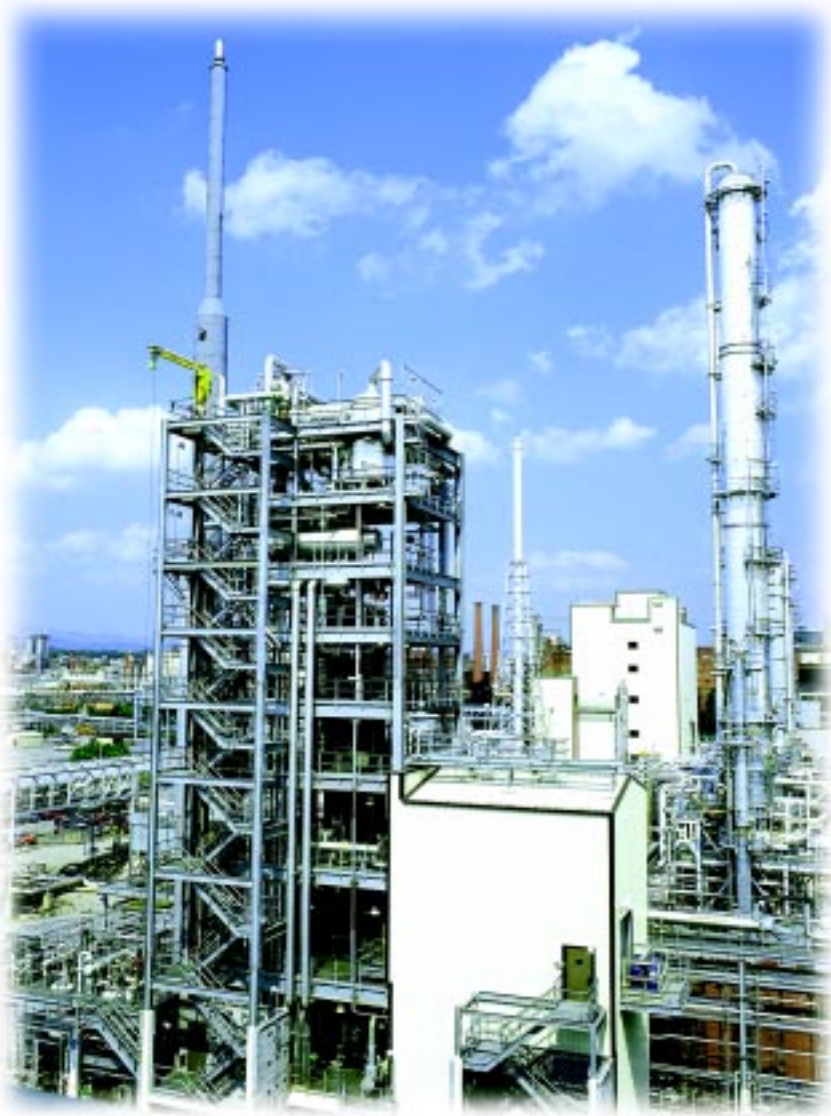
View of LPMEOH™ Demonstration Unit with building housing catalyst facilities in foreground
