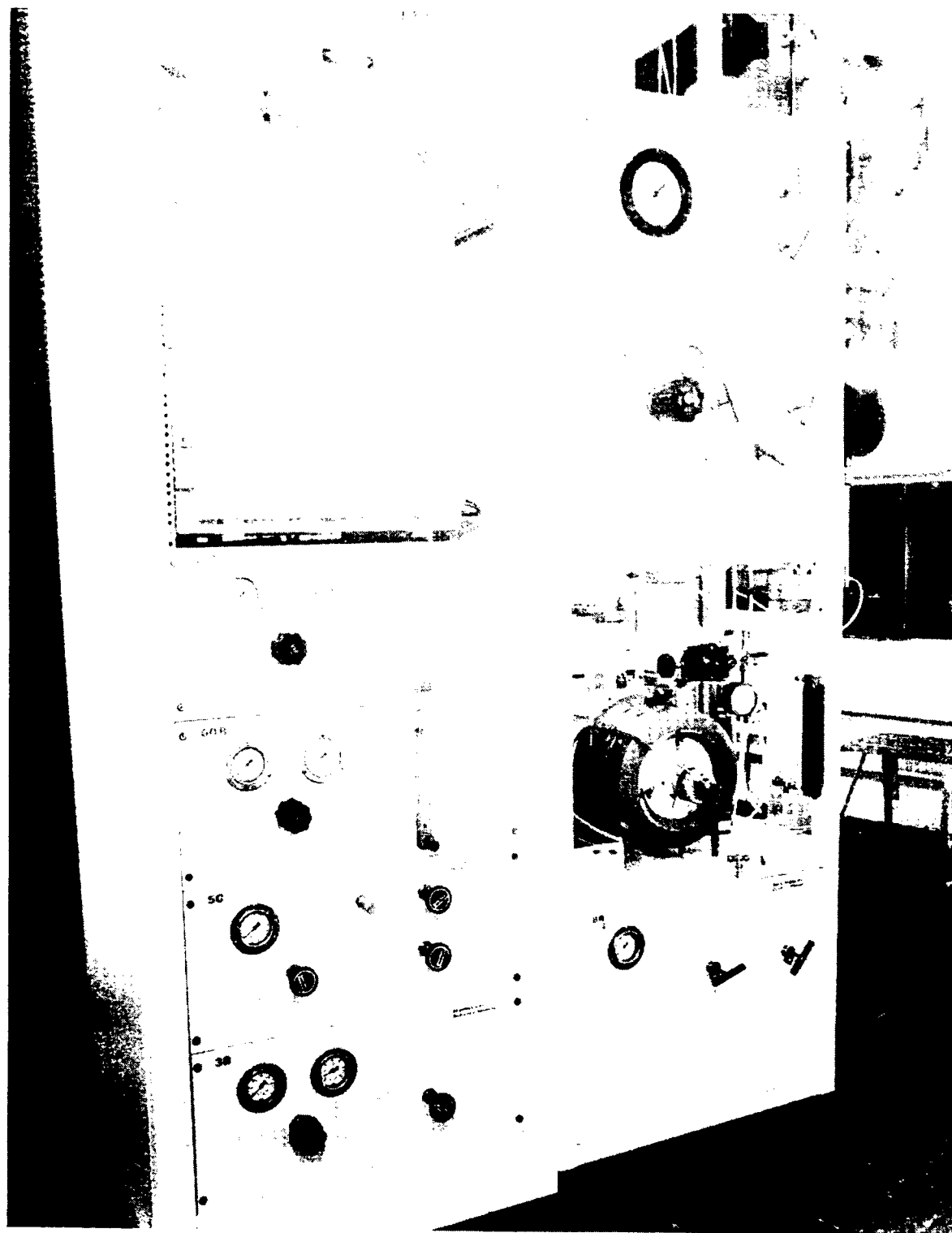
Figure 7. REACTOR CONTROL PANEL
