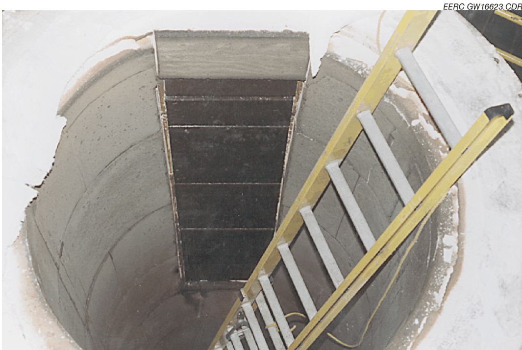
Figure 3-39. Photographs of the RAH panel inside of the slagging furnace following the January (top) and February (bottom) tests.
