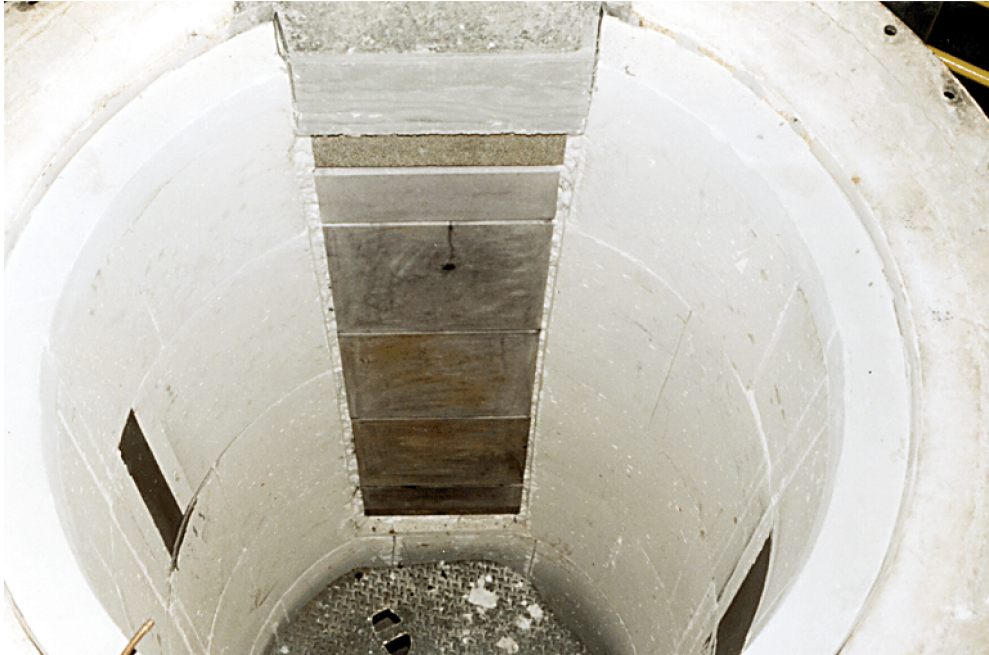
Figure 3-38. Photograph of new ceramic tiles installed on the RAH panel inside of the slagging furnace in January 1999.
