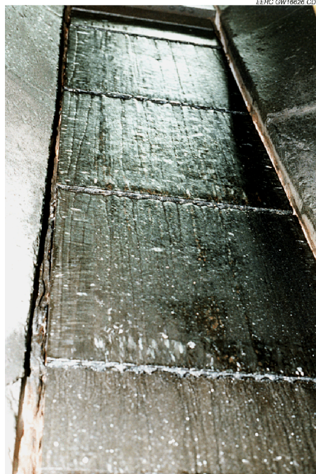
Figure 3-44. Photograph of the RAH panel from inside of the furnace following the April test.
