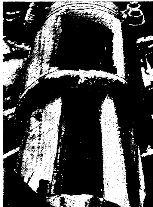
Fig. 6. Photograph of Insulation Removal. Note dual thickness at the cap end of "top tee." Neg. No. MSD-63857.
