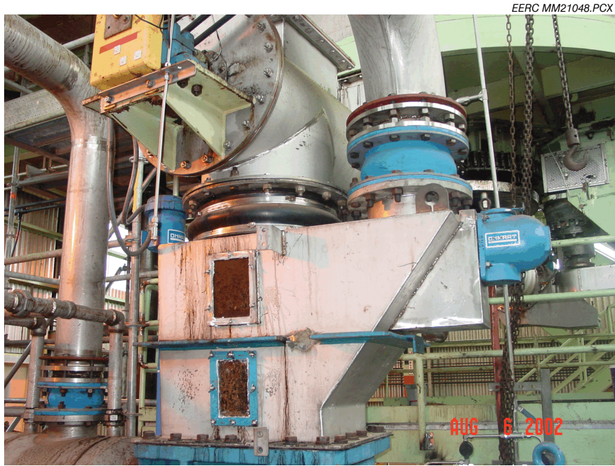
Figure 46. Wood chip-feeding system for plug-screw feeder.
