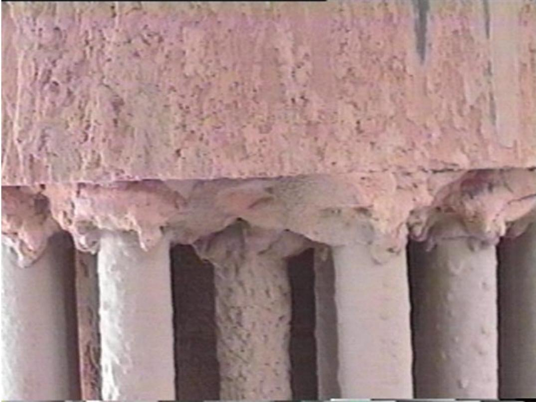
Figure 3-82. This photograph shows the typical ash deposits formed around the mounting locations on the top filter plenum at the PSDF (May 18, 1998).
