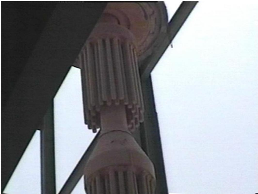
Figure 3-77. Appearance of the entire filter assembly on May 18, 1998 during removal from the filter vessel.
