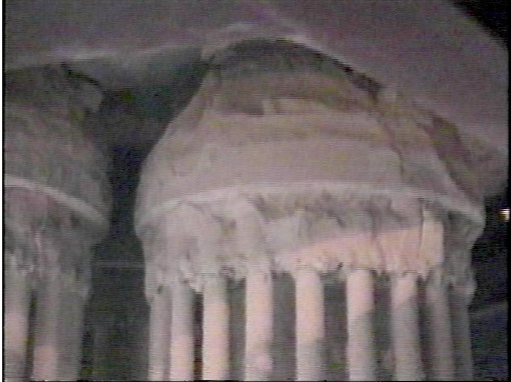
Figure 3-33. Condition of the tubesheet and top portion of the top plenum.
