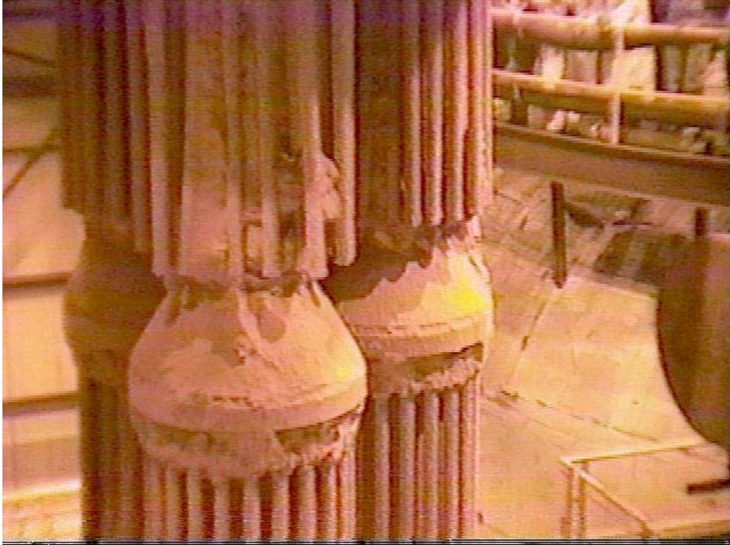
Figure 3-9. Portions of the top and middle plenums are visible in this photograph.
