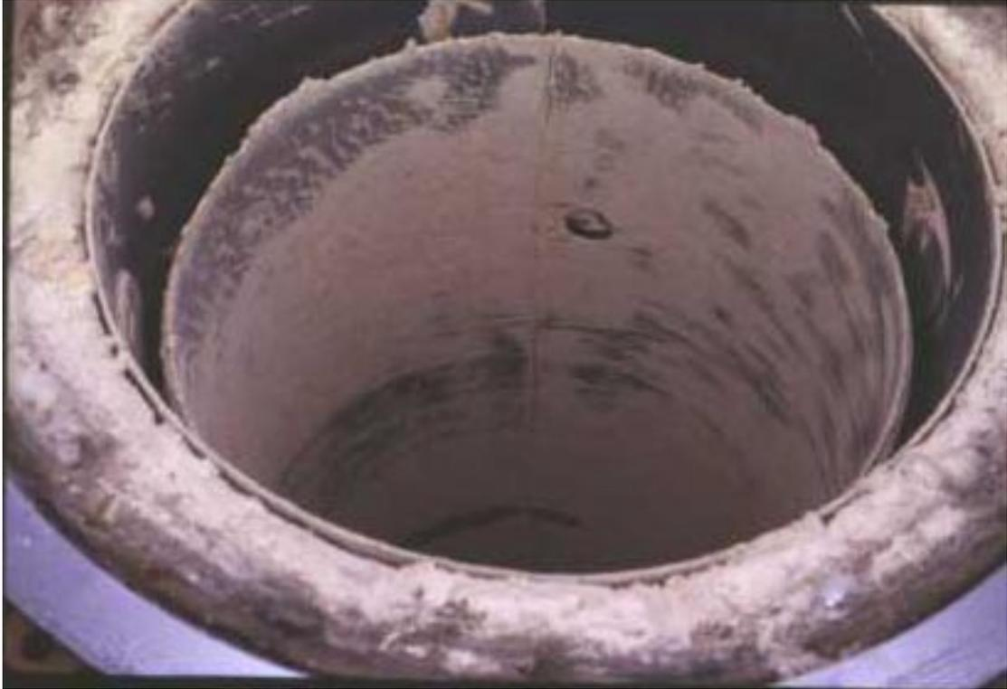
Figure 3-62. Interior of the filter vessel showing the shroud that surrounds the plenums.
