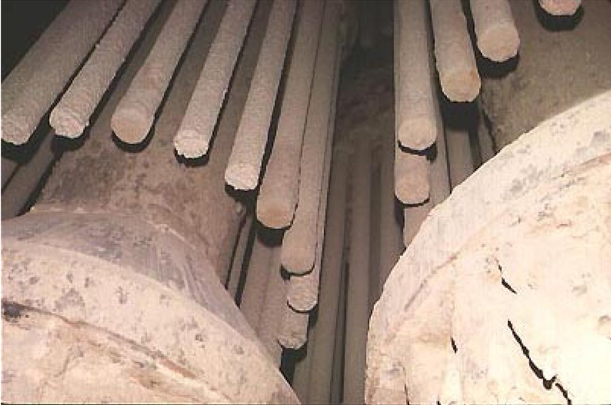
Figure 3-50. The ash sheds and the central support columns remained free of significant ash deposits.
