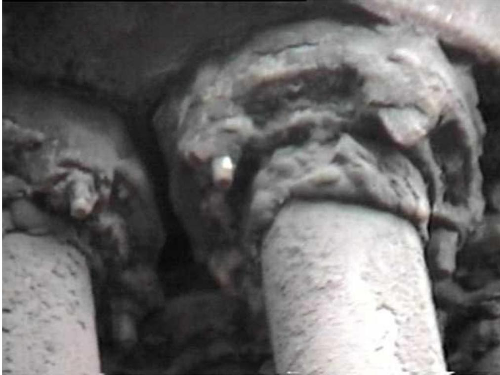
Figure 3-57. Typical deposits that formed around the filter element mounting assemblies.
