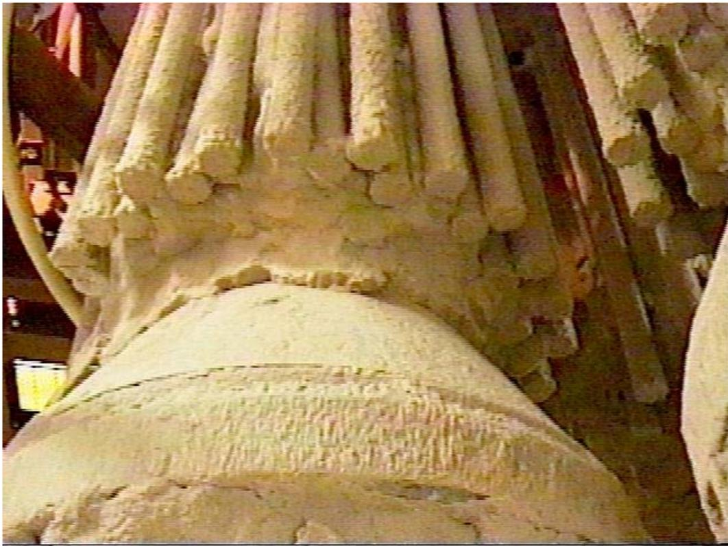
Figure 3-14. Bridging was especially severe adjacent to the central support column.
