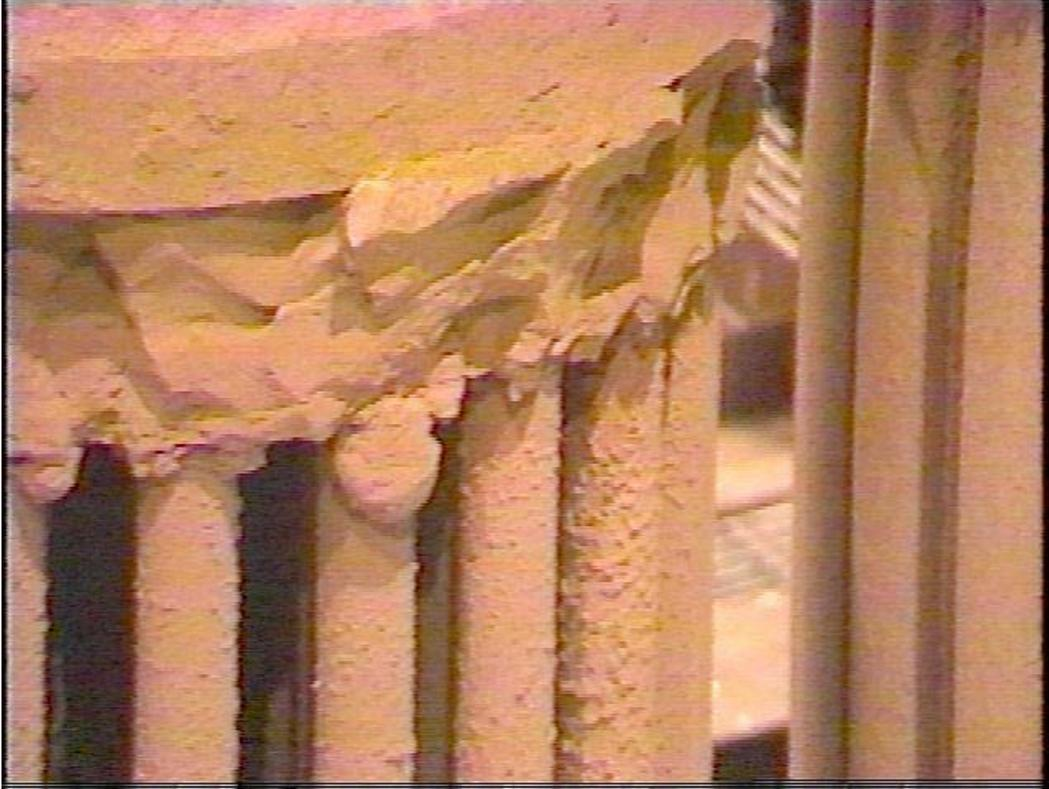
Figure 3-31. View of a tubesheet ash deposit on the bottom plenum.
