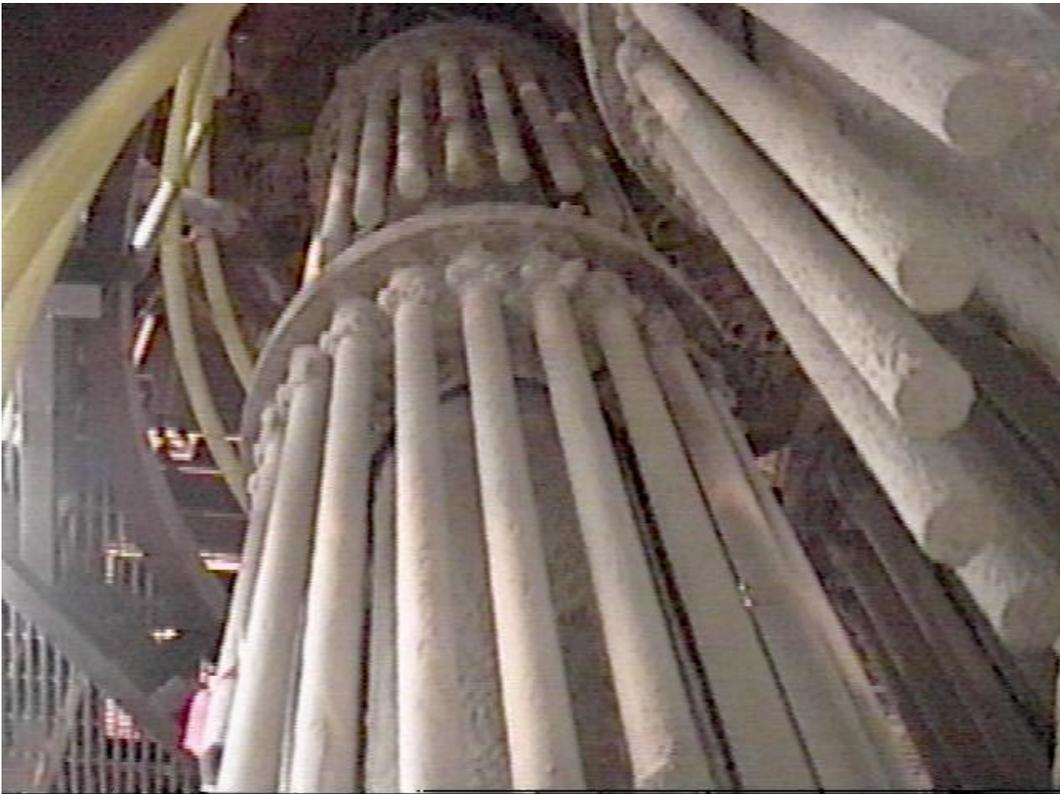
Figure 3-47. This view looking up at the top two plenums shows how the inner ring of elements was removed prior to this run, and how the elements remained relatively clean.
