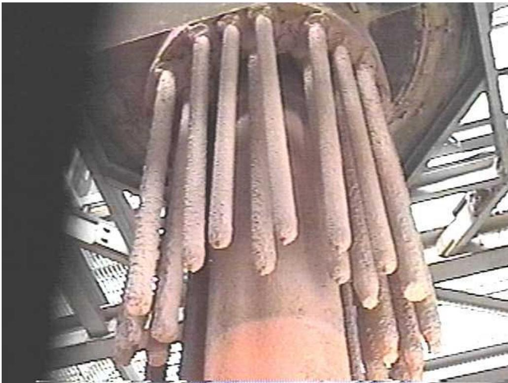
Figure 3-85. Overall view of candles in the top plenum (January 26, 1999).
