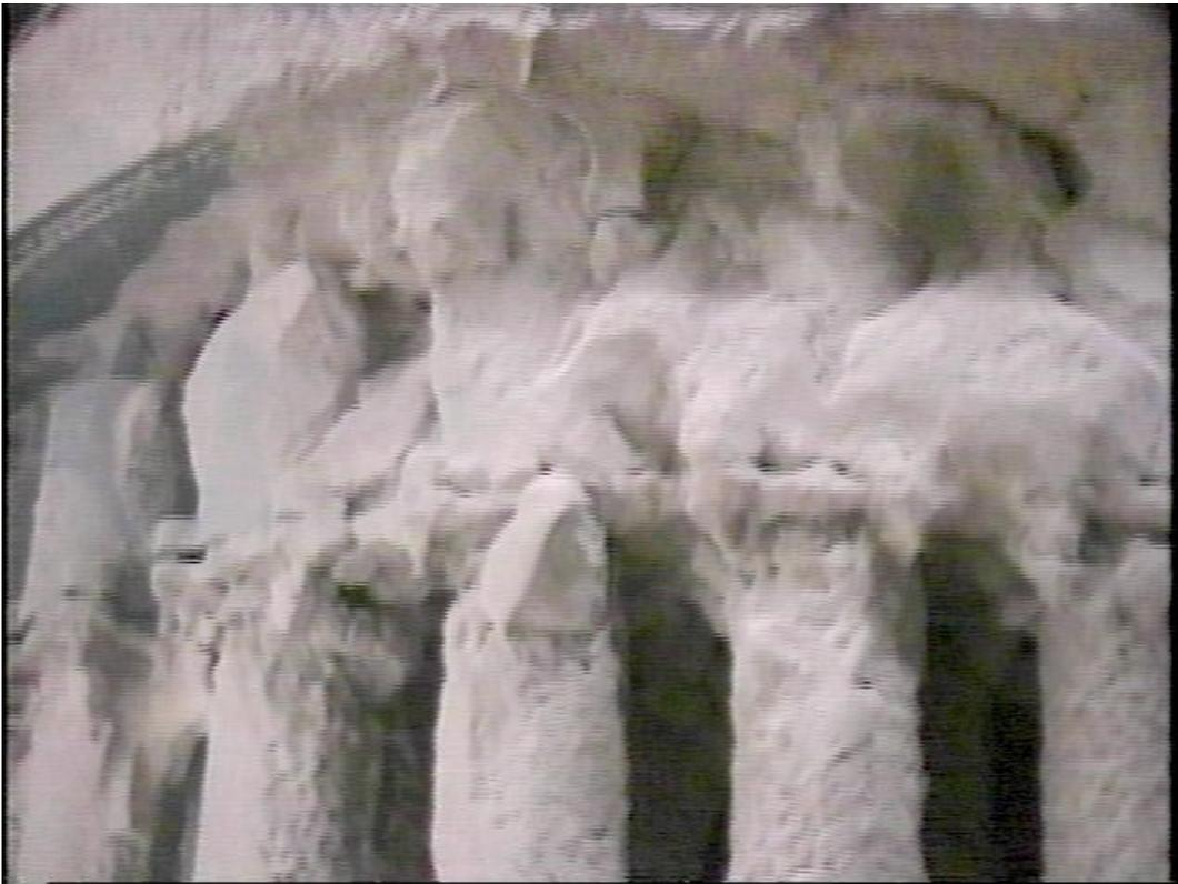
Figure 3-32. View of a tubesheet ash deposit on the top plenum.
