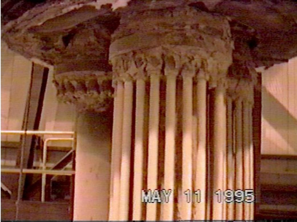
Figure 3-38. Breakages in the plenum on the left were attributed to factors other than ash characteristics.
