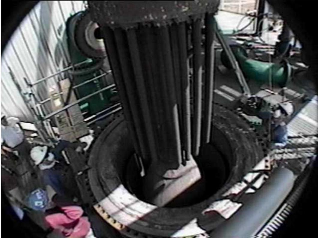
Figure 3-53. Removal of the filter assembly for inspection and refitting.
