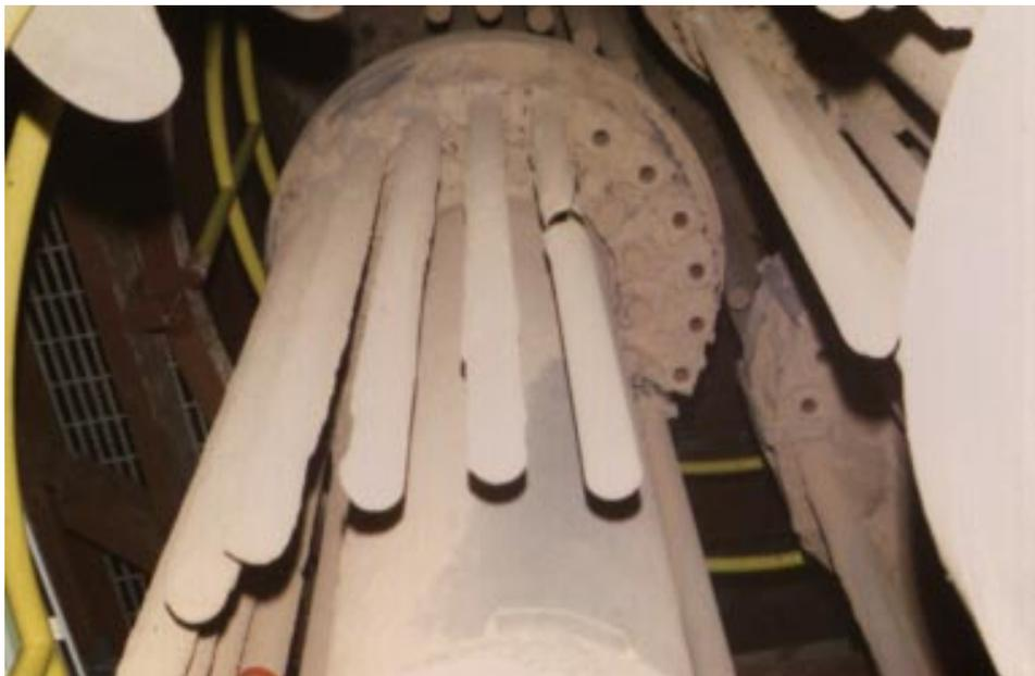
Figure 3-36. This view looking up at the middle plenum shows six candles that broke during operation. The appearance of the central support column suggests that cleaning pulses passing downward through these six locations scoured the column clean.
