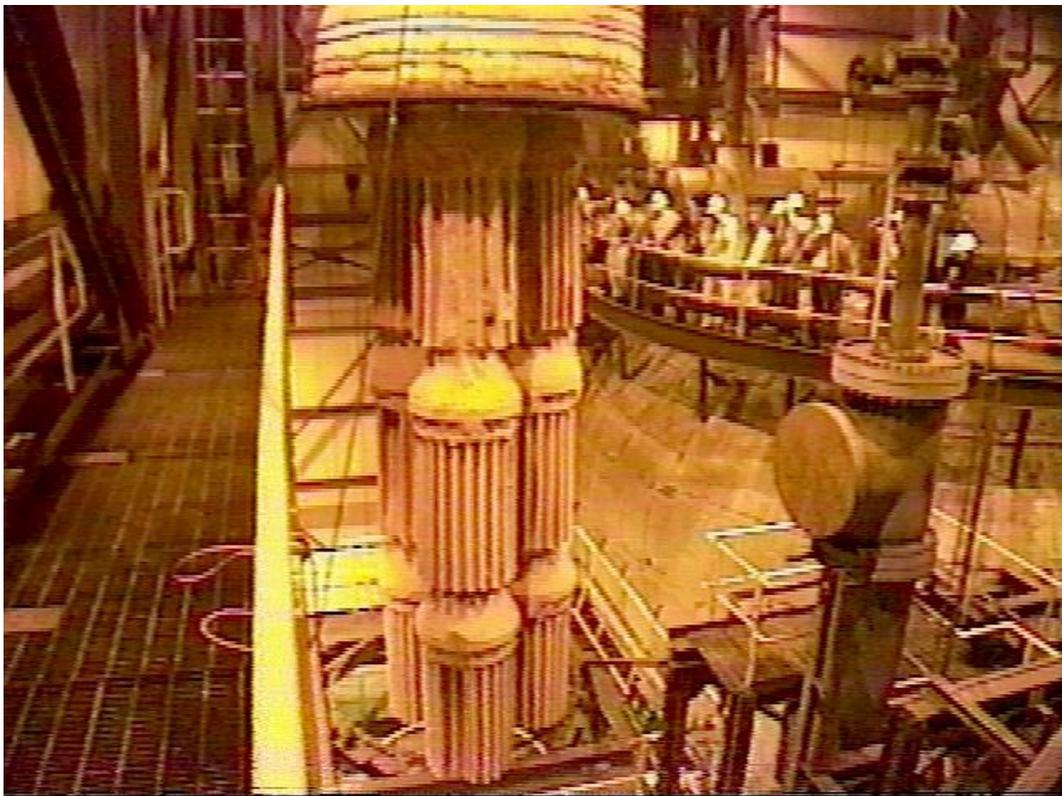
Figure 3-10. The entire plenum assembly being transported to the inspection platform.
