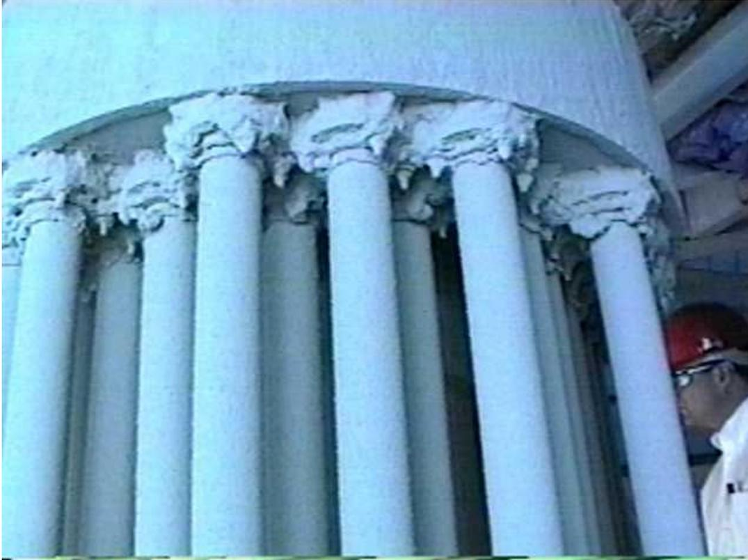
Figure 3-67. Upper portion of filter elements. The blue color in this photograph was caused by blue tarps surrounding the inspection platform.
