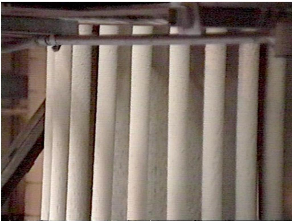
Figure 3-41. The intact candles in the top plenum were very clean.
