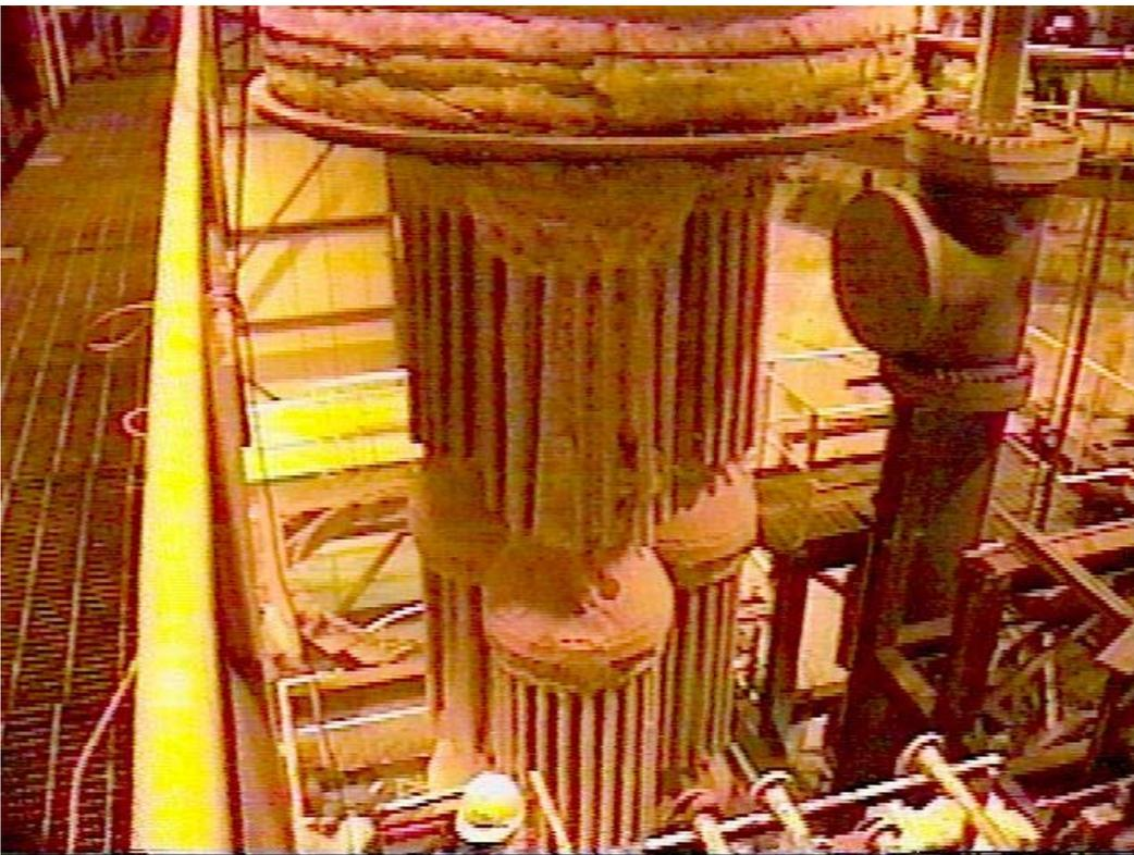
Figure 3-8. A view of the top and middle plenums as the assembly was lifted from the filter vessel.
