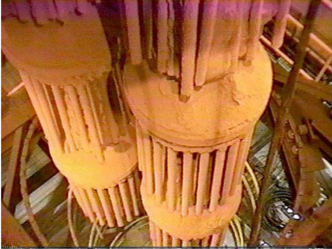
Figure 3-11. Plenums being lowered into the inspection platform.
