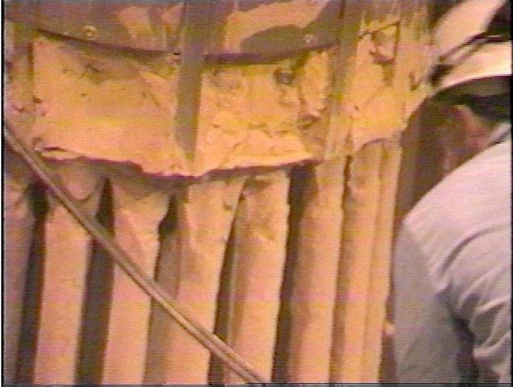
Figure 3-26. This photograph shows a cover that was installed to minimize the growth of ash deposits around the tubesheet.
