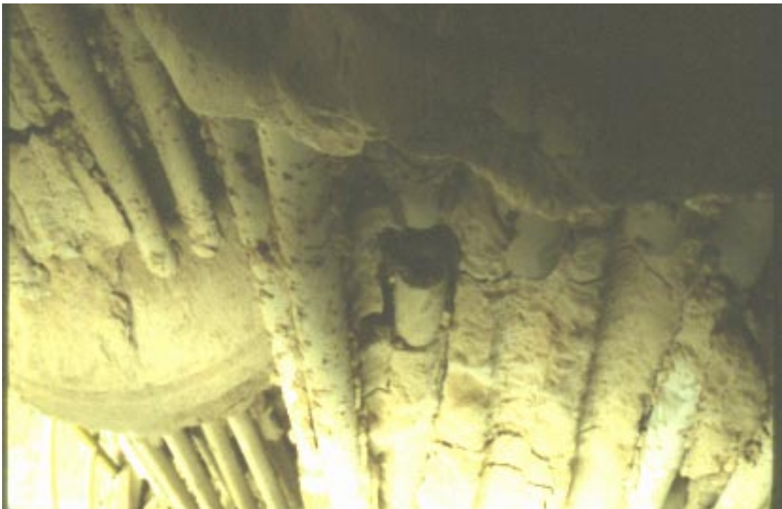
Figure 3-4. Ash almost completely enveloped many of the candle filter elements.
