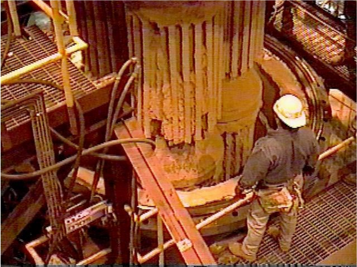
Figure 3-2. Severe ash bridging was evident as the top two plenums were lifted into view.
