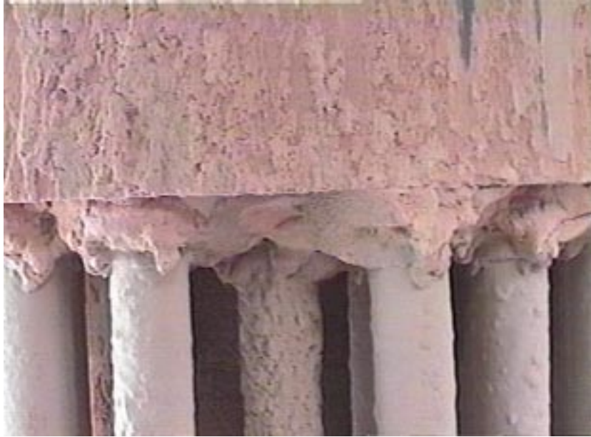
Figure 8. This photograph shows the typical ash deposits formed around the mounting locations on the top filter plenum (May 18, 1998).
