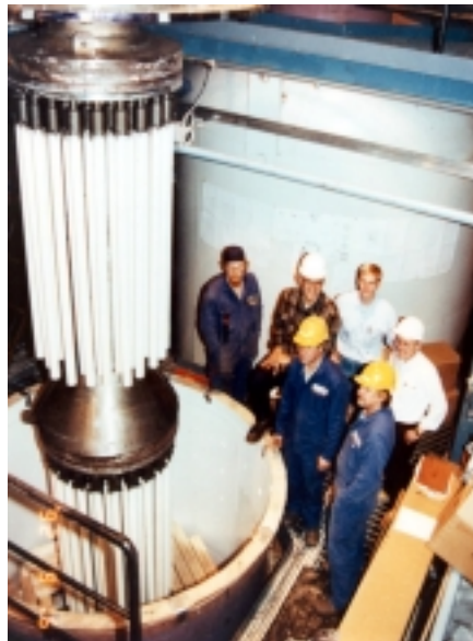
Foster Wheeler PCFBC Facility
