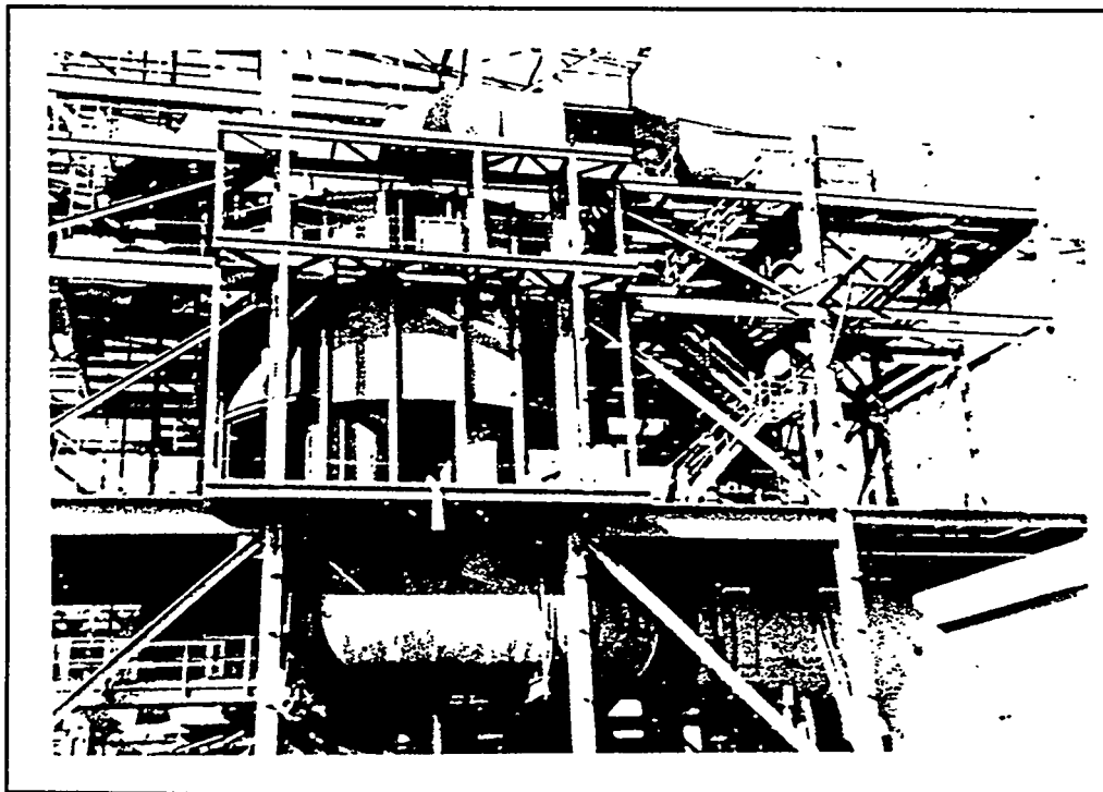
Figure 8.21 Dryer, Inlet Duct and Outlet Duct
