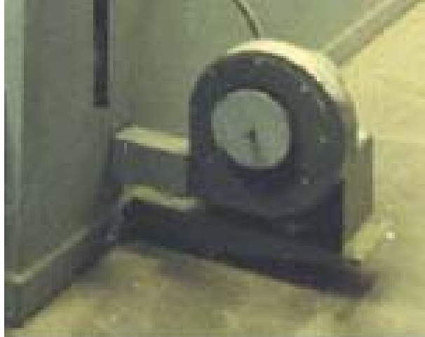
Figure C-11. Under fire fan assembly
