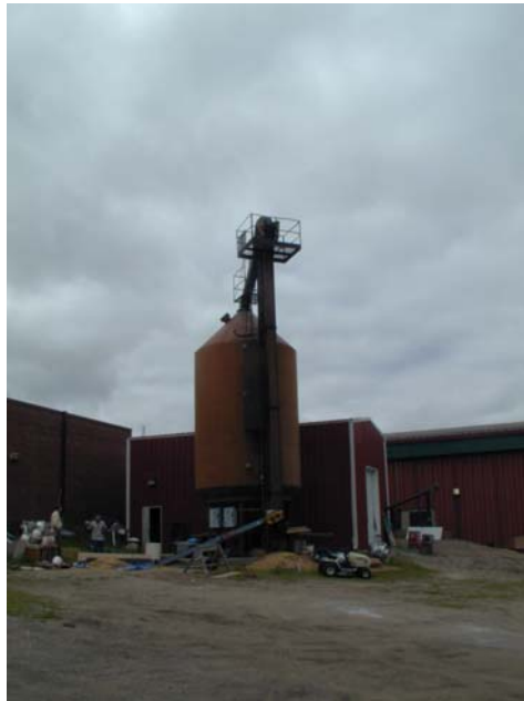
Figure 4-3. Pellet Fuel Hopper for Humanities Building
