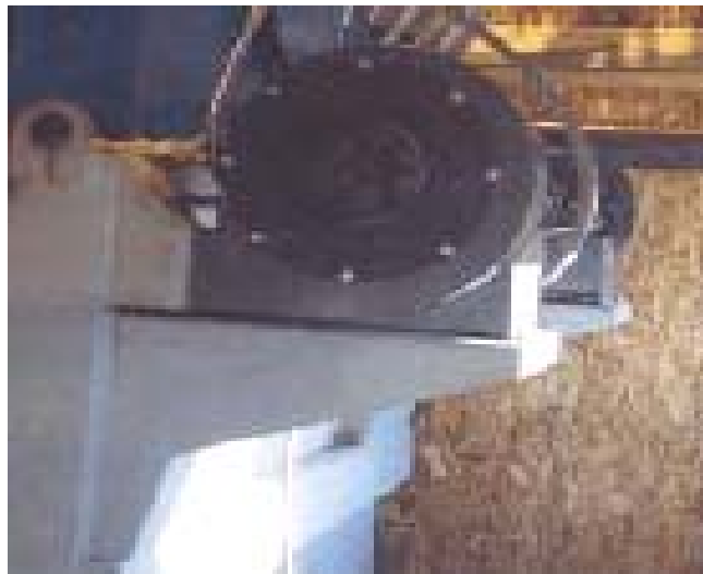
Figure C-12. Over fire fan assembly
