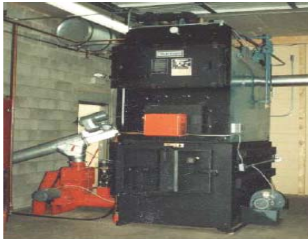
Figure C-10. Integrated Combustor/Boiler Configuration
