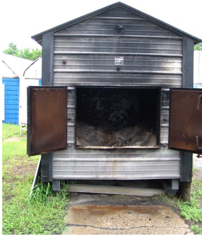
Figure 4-4. Biomass Boiler at Forestry Division Tree Seedling Greenhouse, Redby, MN
