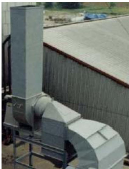
Figure C-13. Representative Exhaust Stack
