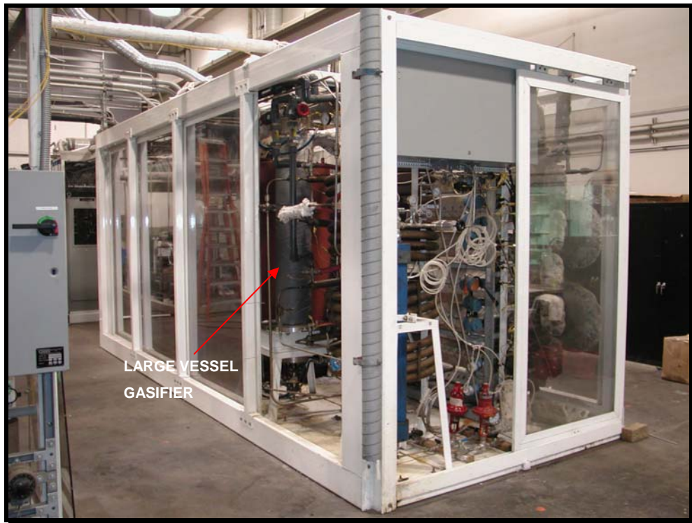
Figure 2-4. SWPO reactor skid with shielding and large vessel gasifier installed.
