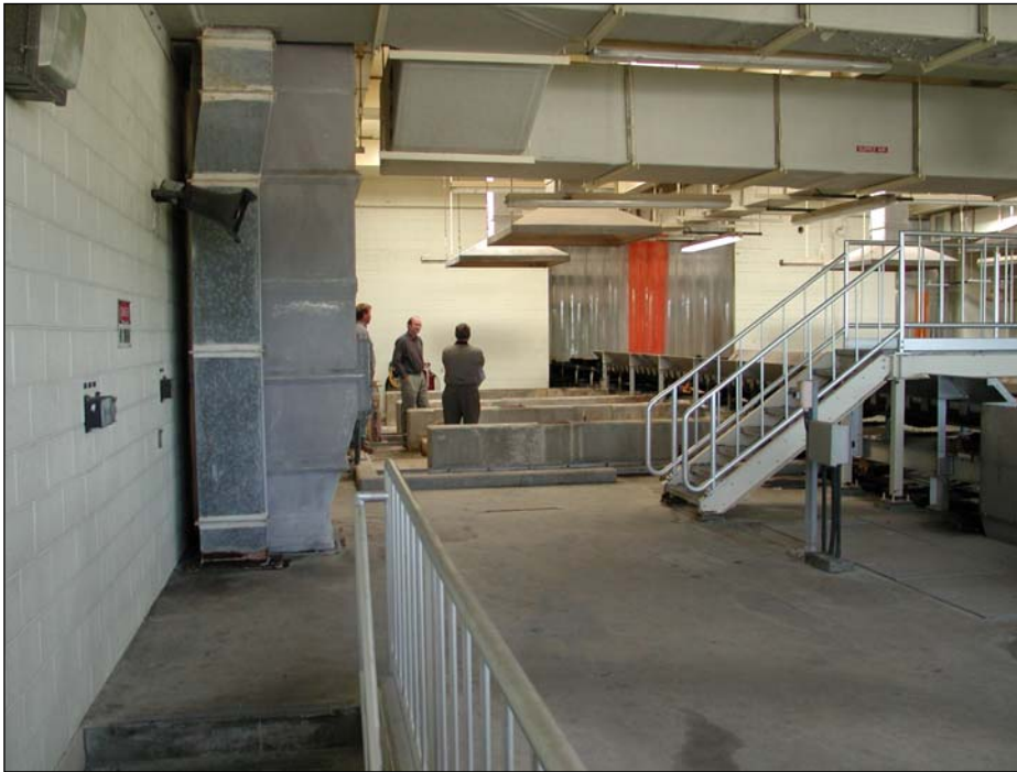
Figure 4-6. Encina sludge conveyor room is available for a SWPO reduced-scale demonstration unit.
