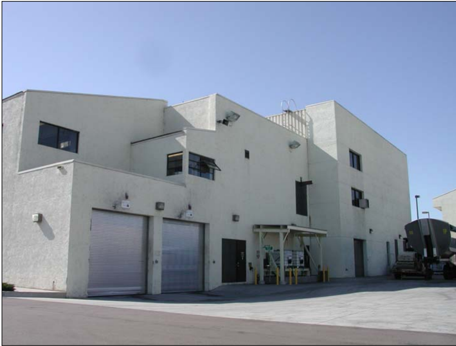
Figure 4-5. Encina sludge dewatering building, a potential SWPO reduced-scale demonstration site.
