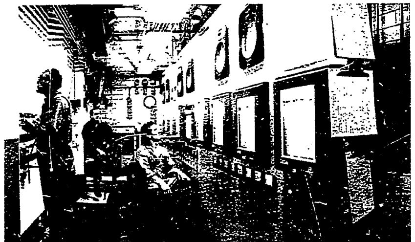
Figure 5. Control center for the 1/5 ton per day liquefaction pilot plant. Operating conditions throughout the plant are monitored on the panel at right. At left are manual controls which extend through the safety wall and allow adjustment of flows in the high pressure plant area.
