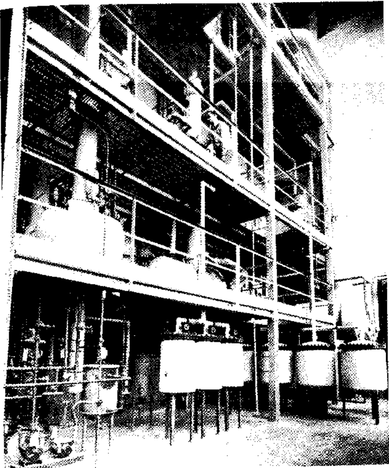
Figure 41. - Batch-distillation equipment (100- to 500-gallon).
